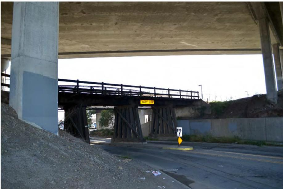
Photo 13: Existing trestle over Woodland Avenue/Bellam Boulevard. U.S. 101 crosses over the alignment at this location. The trestle would be replaced as part of the Proposed Action.
