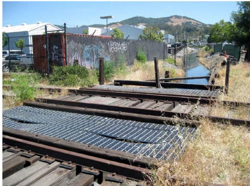
Photo 9: Existing trestle across unnamed channel between Rice Drive and Andersen Drive. This structure would be replaced as part of the Proposed Action.
