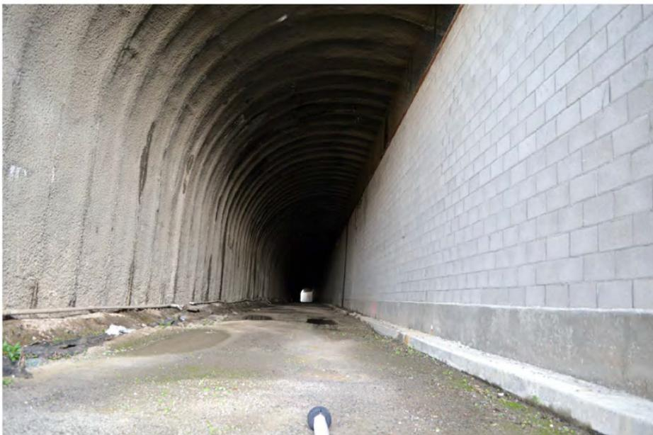
Photo 17: Interior view looking north within the Cal Park Hill Tunnel of the SMART ROW. Masonry wall to right separates the SMART ROW from the Cal Park Pathway.
