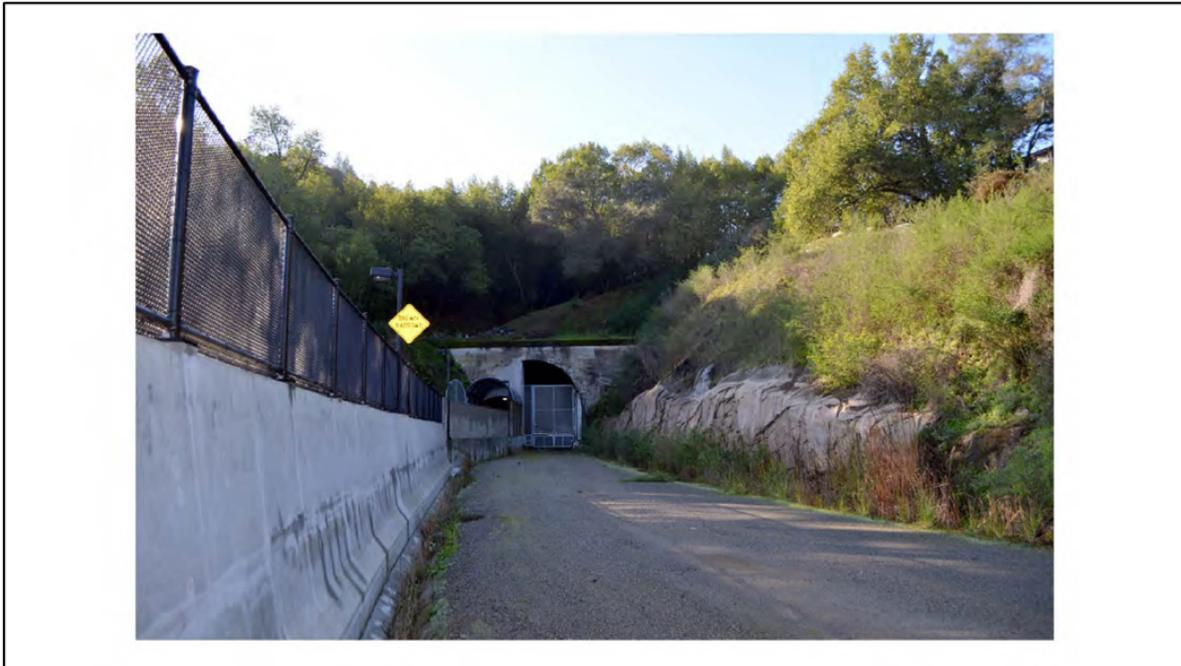
Photo 15: View of the alignment looking south at northern portal of the Cal Park Hill Tunnel. SMART ROW occupies the right side of the tunnel, the Cal Park Pathway occupies the left side.
