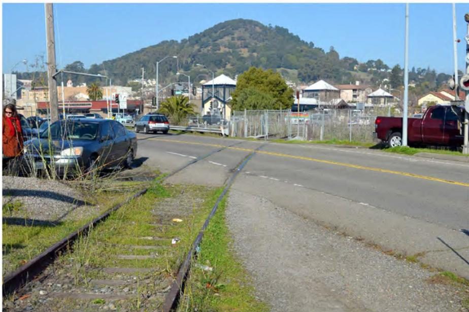
Photo 6: View of alignment looking north across West Francisco Boulevard. This crossing would be eliminated as part of the Proposed Action by flipping the location of the roadway relative to the tracks.
