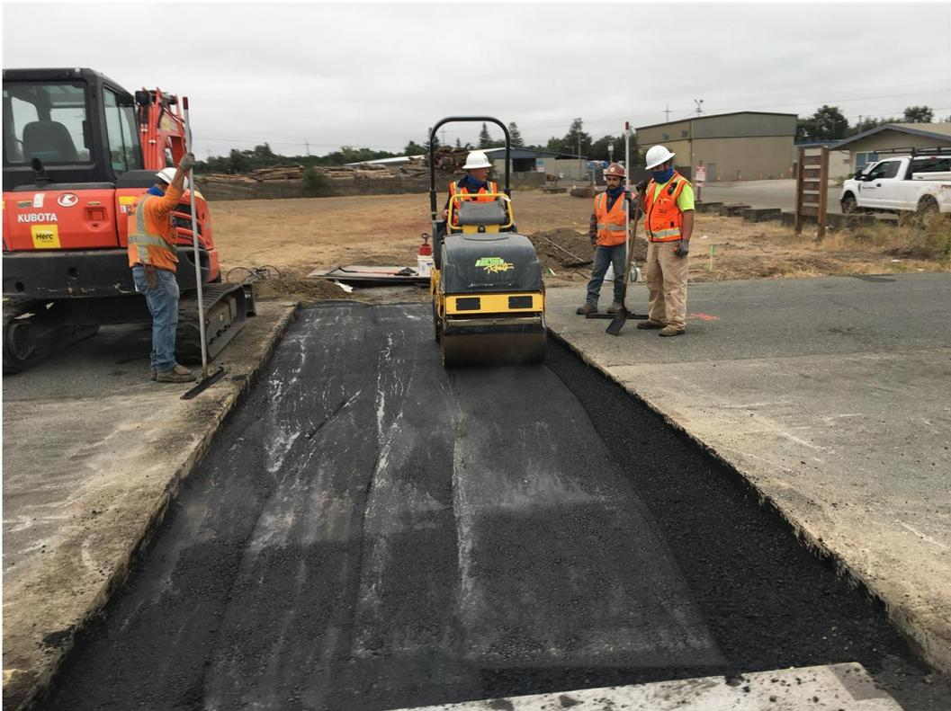
*Airport Blvd.- Pavement Restoration After Drainage Culvert Installation*
