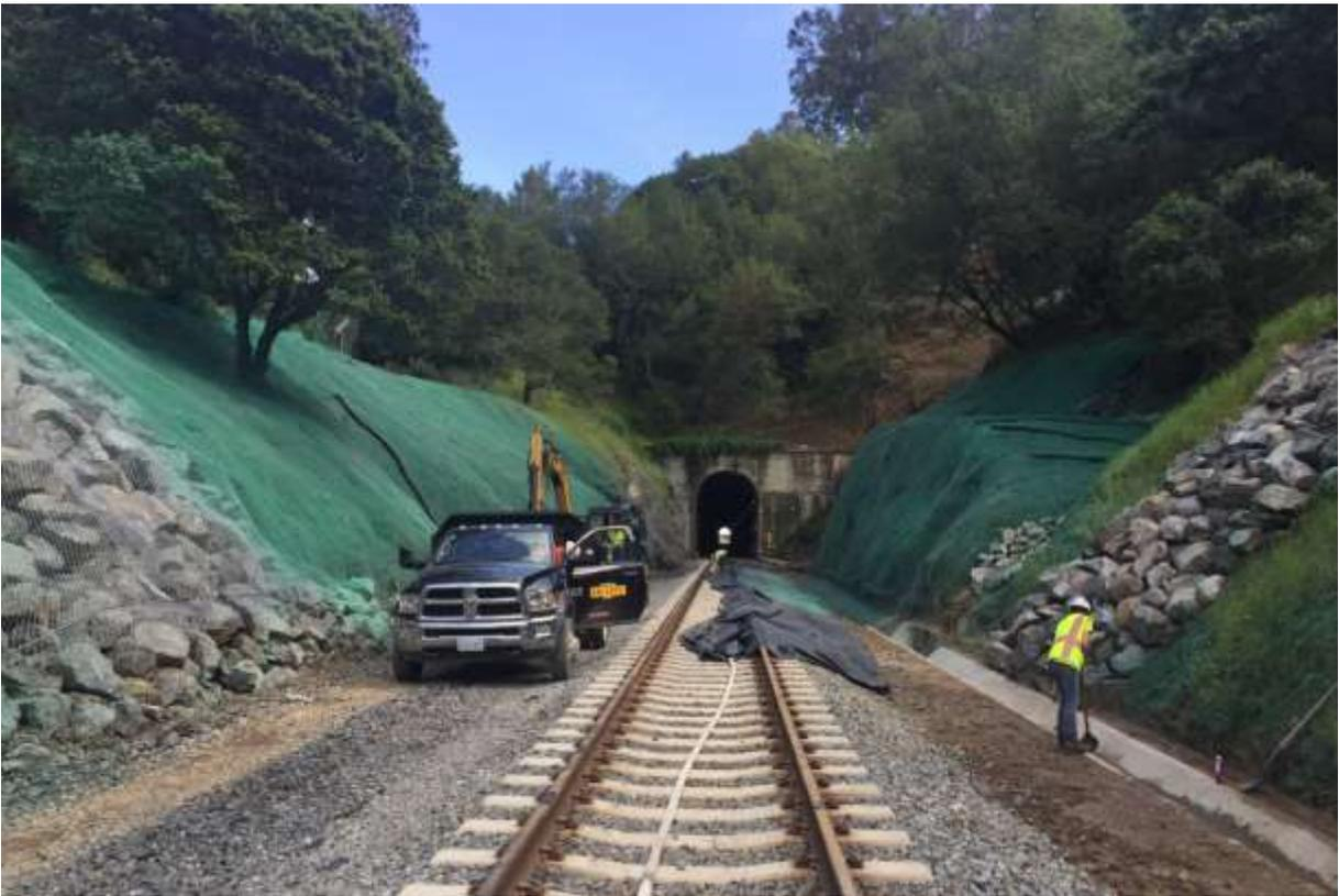
View of the Puerto Suello tunnel's northern entrance after the newly shaped slopes have been hydro-seeded.
