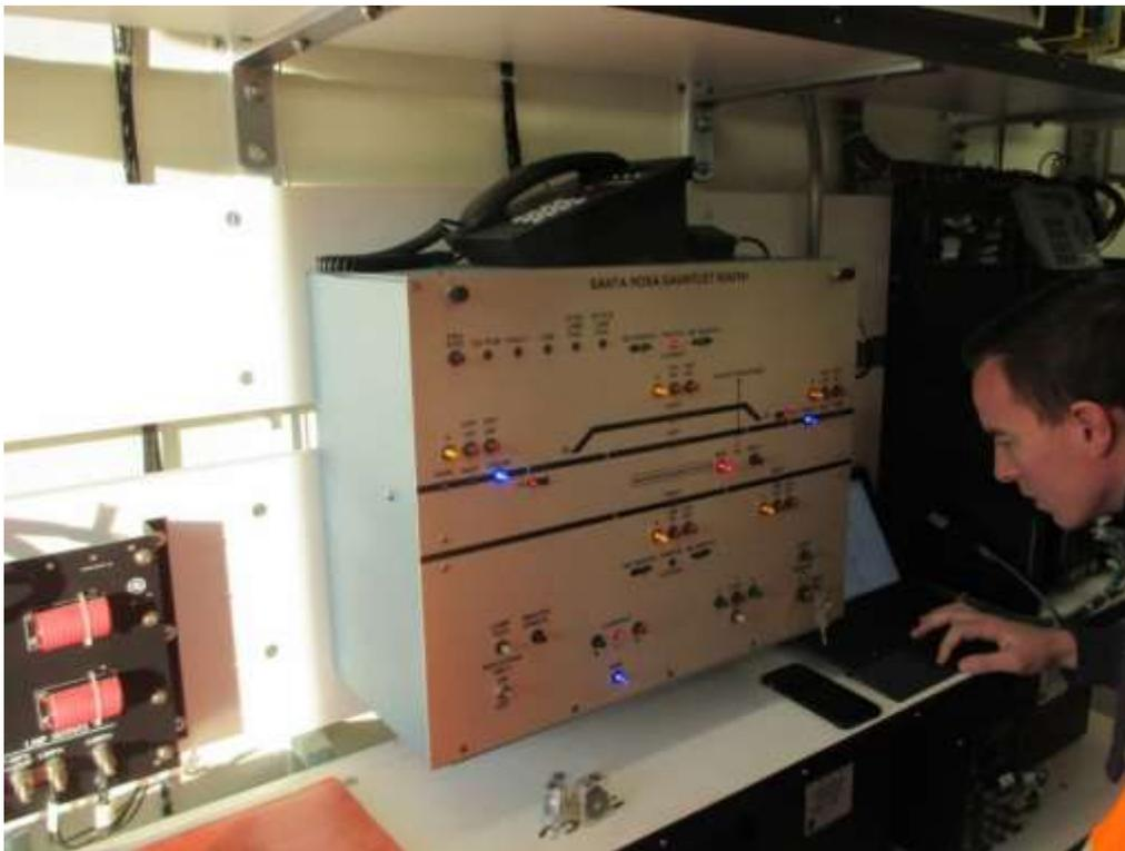
Signal Engineer verifying vital processor setup during testing, Santa Rosa
