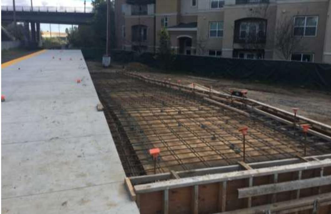
Ramp rebar finished and ready for deck pour at south of station.
